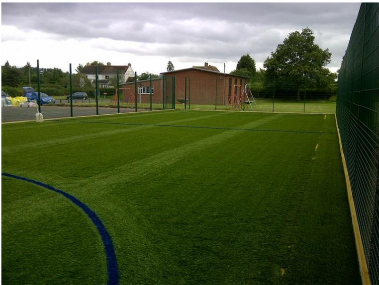
The maintenance of long pile artificial grass is similar to that for sand-filled, taking into consideration the longer pile and rubber infill. If maintenance is not carried out, performance quality will deteriorate and the life of the carpet will be reduced. Guarantees may also be affected.
